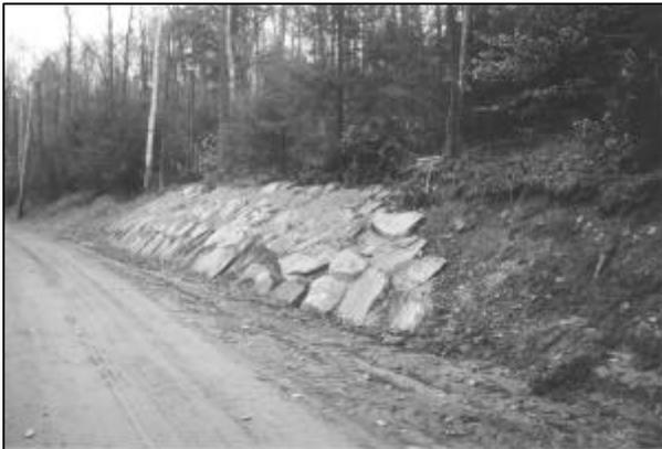
3. A Work in Progress: To stabilize the bank, the town used a combination of small and large rocks on the face of the bank. A ditch was constructed along the toe of the slope and culverts were used to direct runoff to stable outlets before it reached the river.
