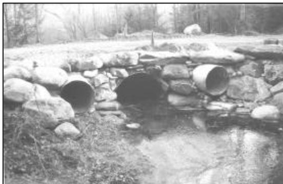
3. Headwalls and endwalls were constructed using stone found on site. The new culverts are expected to adequately handle heavy flows, thereby improving the protection of the road.
